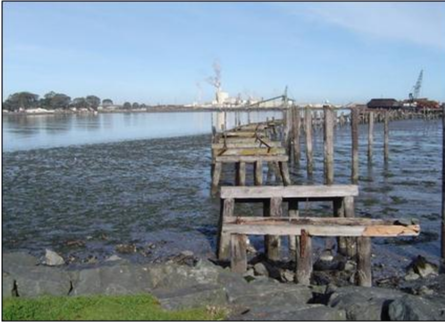
Figure 6.10. Pilings Supporting an Abandoned Trestle in Humboldt Bay, California.
